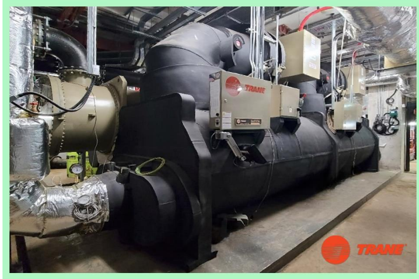
The 2,200-ton Trane® Duplex™ CenTraVac® chiller @HFO R514A
